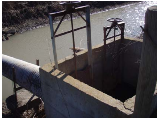
Set of Watergates in a Vault South of Swan Road
