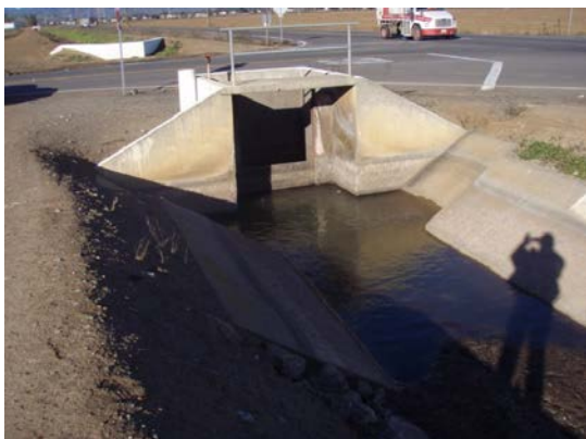
Flashboard Risers in a Box Culvert at the Southwestern Corner of the Fry Road and Meridian Road Intersection
