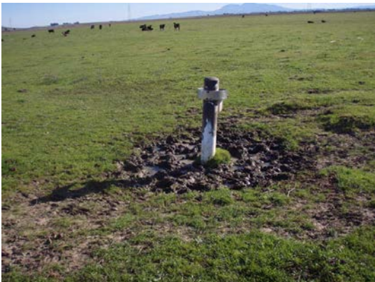
Cathodic Protection Station, South of Cordelia Road and West of Pennsylvania Avenue
