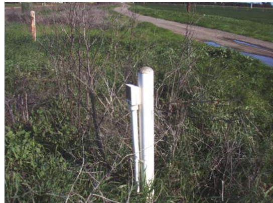
Cathodic Protection Station, South Side of Cordelia Road and East of Chadbourne Road
