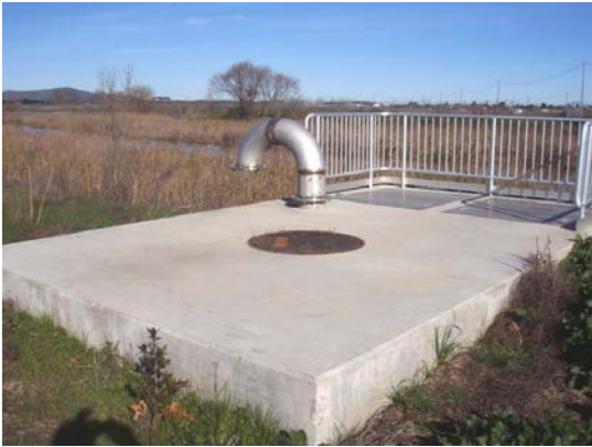
Air Vacuum Relief Valve, North of Cordelia Road on the West Side of Ledgewood Creek
