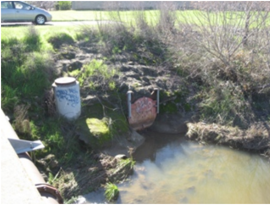
Storm Water Pipe Outfall into Lynch Canyon Creek, City of Fairfield (IMG_1719.JPG)
