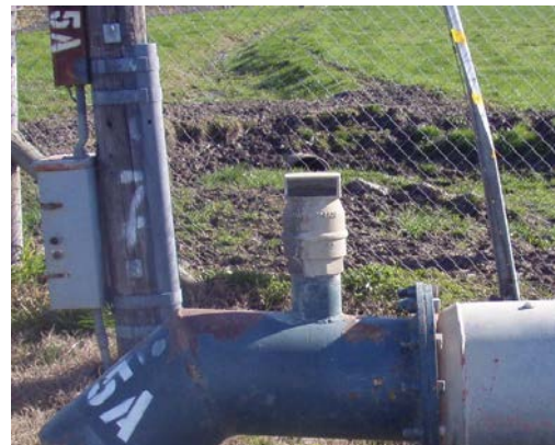
Water Meter on Pump Station 75A, Along Robben Road, North of Binghamton Road
