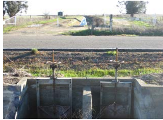
Check on Irrigation Supply Ditch, Solano Irrigation District Facility 25288 (IMG_1756.JPG)
