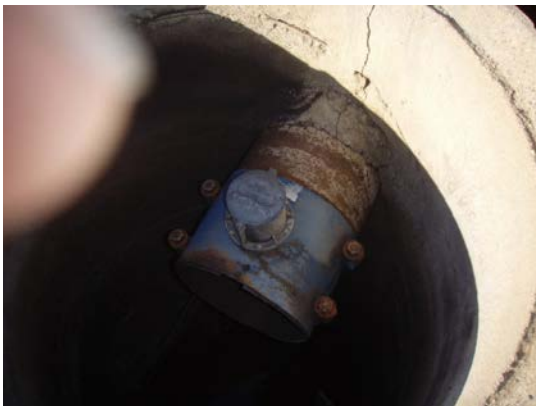
Water Meter in an Upright Culvert Vault on the East Side of Hwy 113 North of Fry Road
