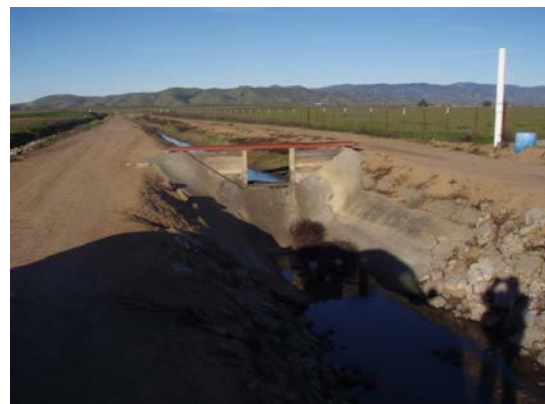
Flashboard Risers, South of McCrory Road, West of Meridian Road
