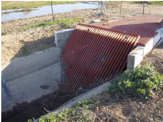
Screens Covering an Inlet at the Northwest Corner of the Intersection of Northgate Road and McCrory Road
