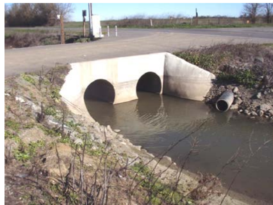
The Headwall of a Set of Culverts Under an Access Road Crossing Located on the West Side of Hwy 113, North of Fry Road
