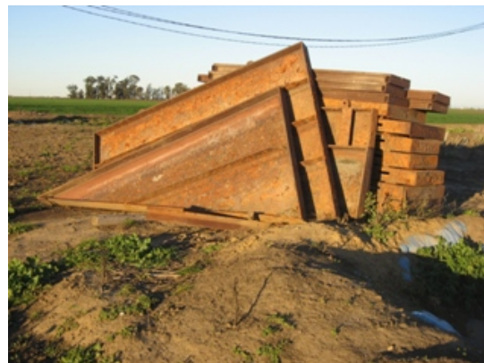
Seasonal Dam 2 Moveable Structure Components Stored During Winter, Maine Prairie Water District (IMG_1772.JPG)
