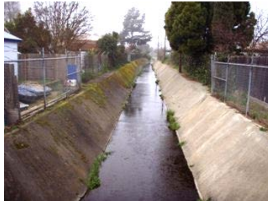
Concrete-lined Storm Water Drainage Ditch, City of Vallejo Sanitation and Flood Control District Facility (P1280370.JPG)
