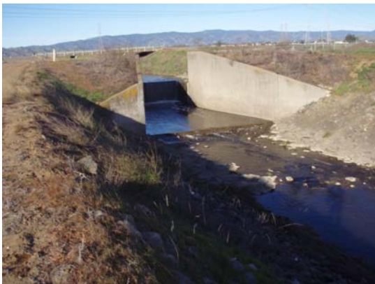
Drop Structure in a Drainage Channel East of Meridian Road and South Of Fry Road
