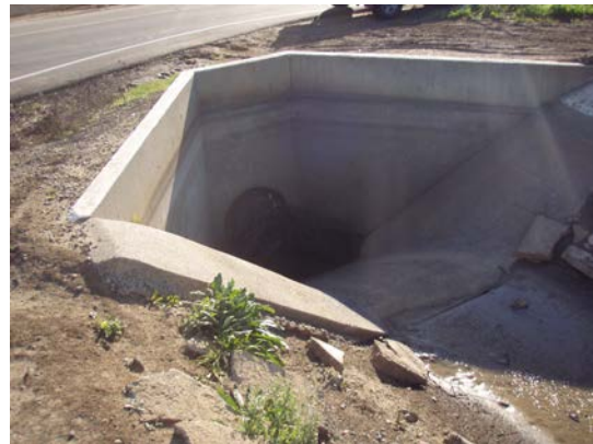
Drop Structure to a Culvert under Meridian Road Just South of Fry Road
