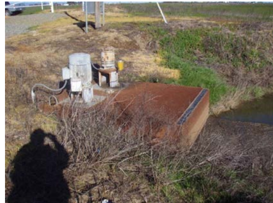
Screens Covering an Outlet Located Along the East Side of Hwy 113, North of Fry Road
